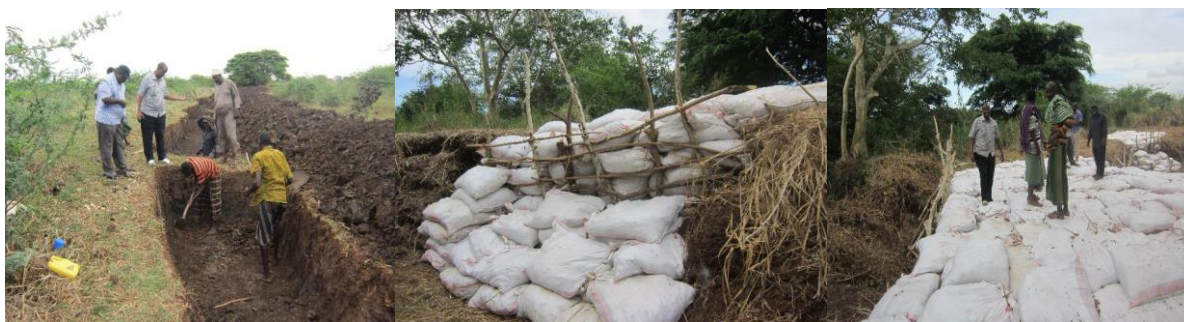
Rehabilitation of Madingo water pan
